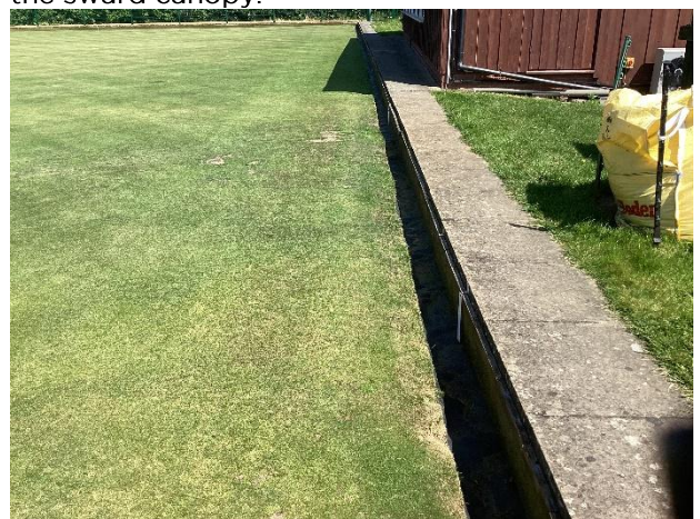
Photo 10: Collapsed edging will impact both play outcomes and plant health outcomes.
